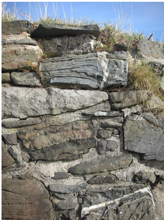
Re-pointing below drainage chute on SW tower wall
