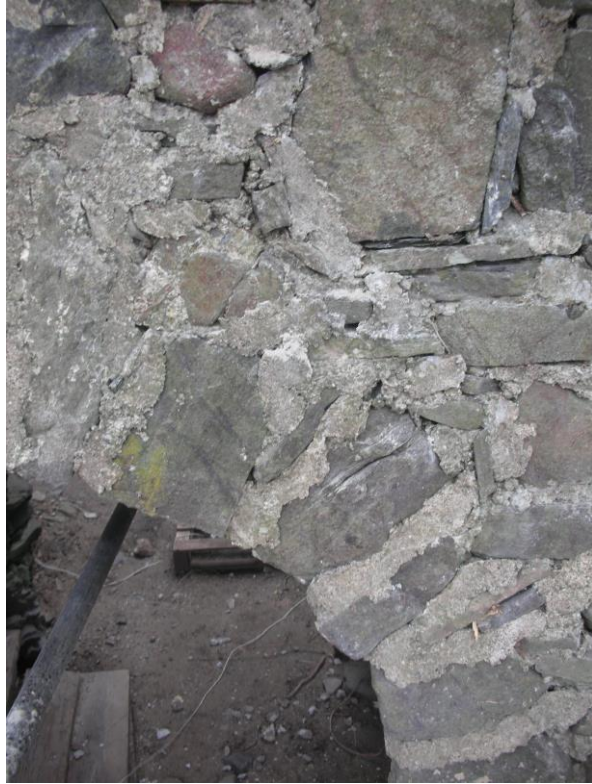
Repair around second floor window in SW tower wall
