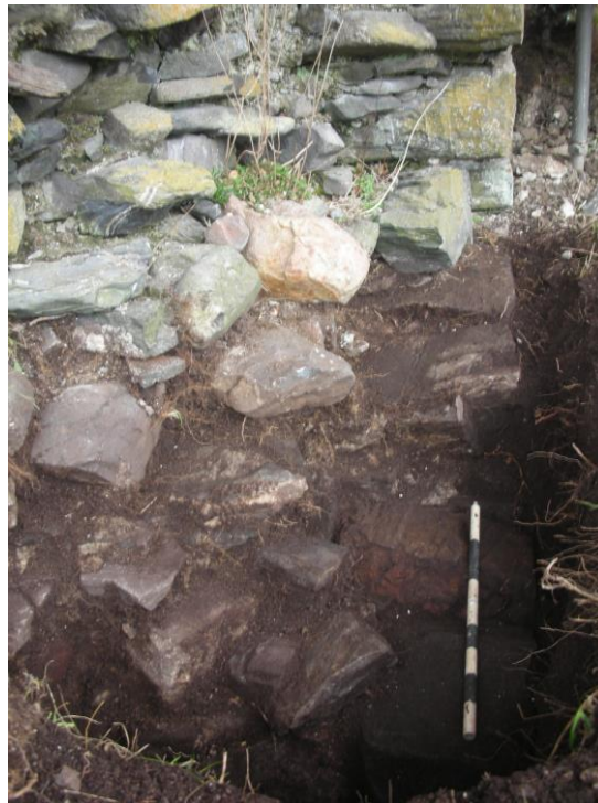
The cleared stonework prior to underpinning
