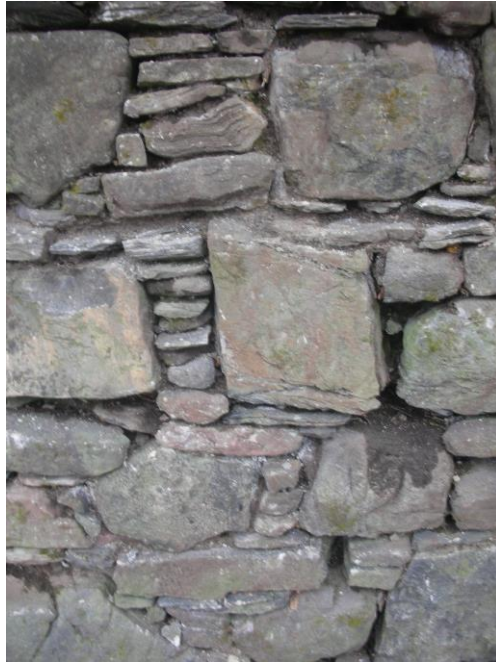
Stone work on tower
