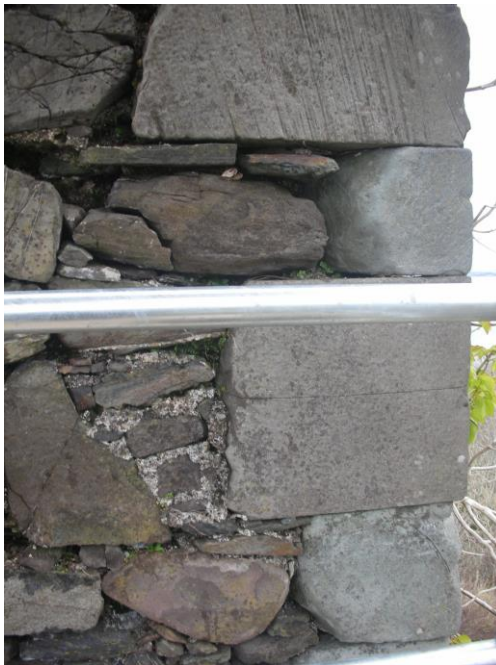
Surviving quoins on SE corner of tower
