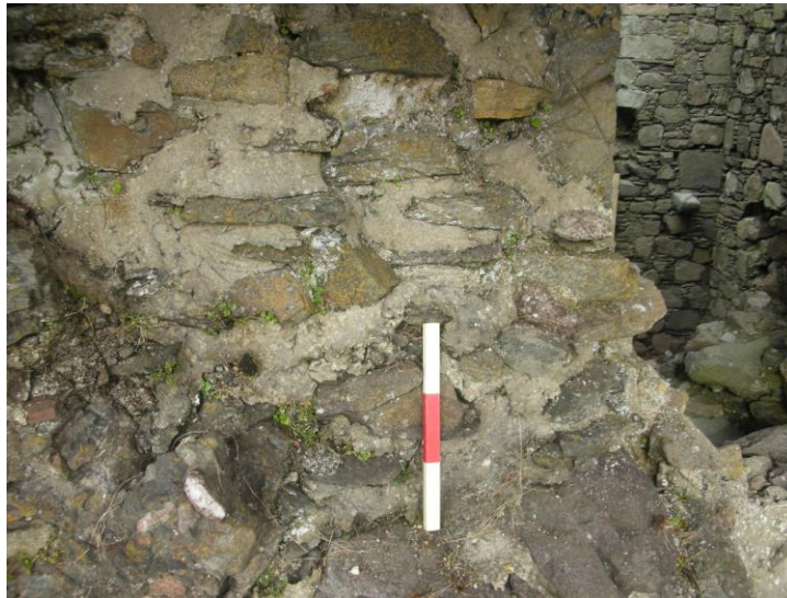
Re-pointing around 2 nd floor window on SE side of tower
