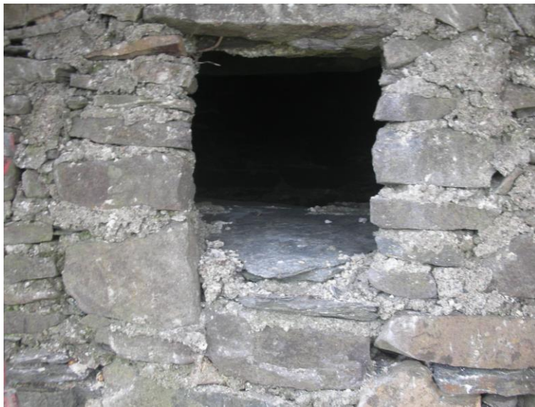
Render repair on upper stair window in SW tower wall
