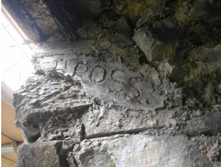
Personalised repair on the first floor entrance
