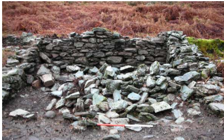
Rubble collapse [002] at east of Structure 2
