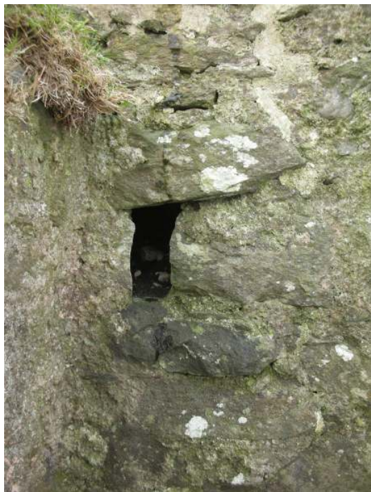
Outwork gun-loop (K) external
