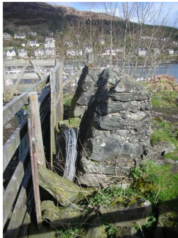
Buttresses of enclosure wall [030]
