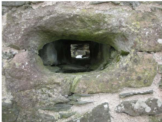
Outwork gun-loop (I) external
