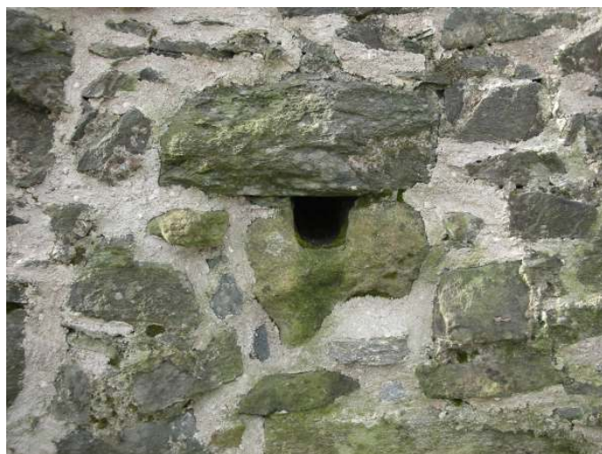
Outwork external drain (L)
