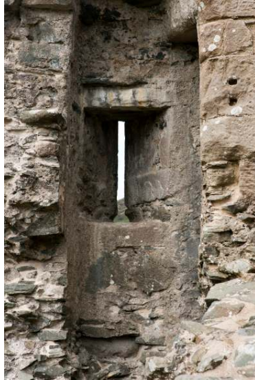
Stair gun-loop (B) internal
