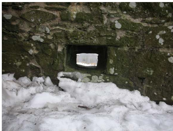
Outwork gun-loop (I) internal
