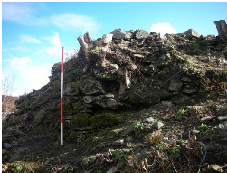
Drum tower [002] external wall
