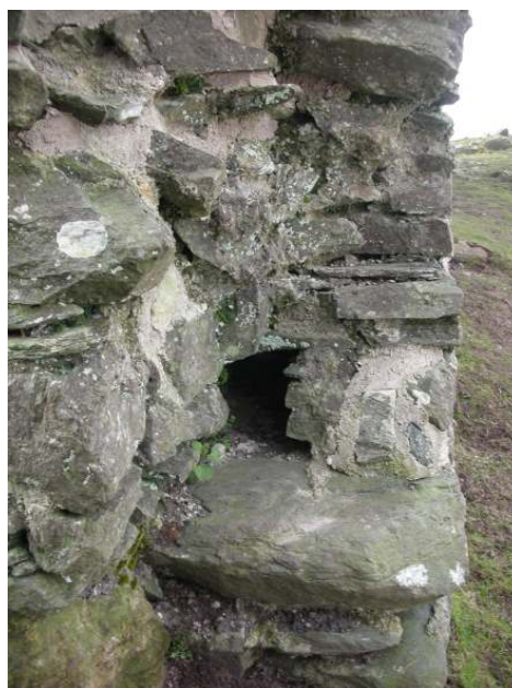
Outwork entrance bare-hole (J)
