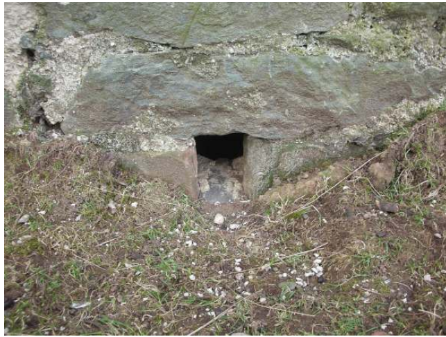
Cellar window (G)
