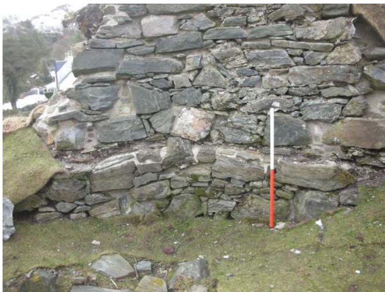
Scarcement in drum tower
