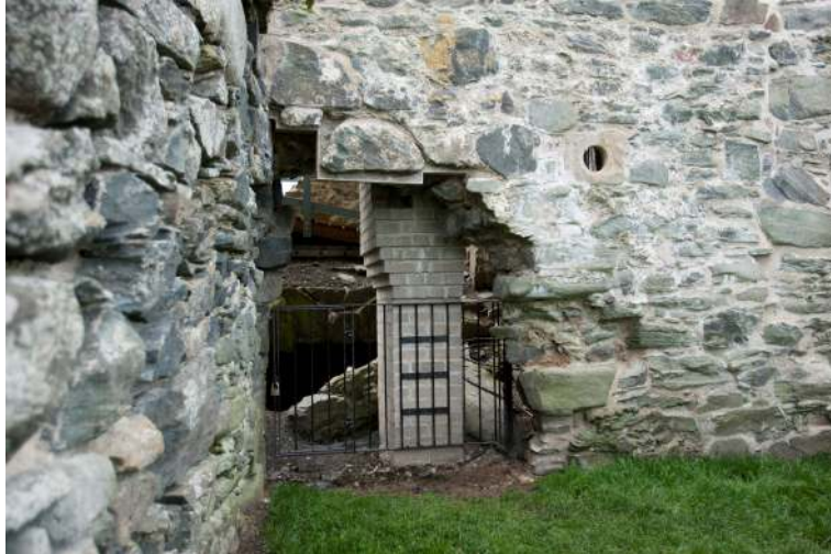
Tower Entrance (F)
