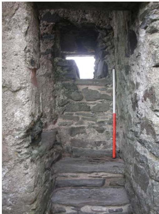
Stairs and blocked window (M)
