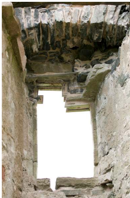
Window (P) internal
