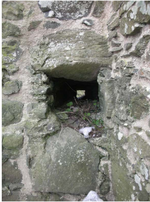
Outwork gun-loop (H) internal
