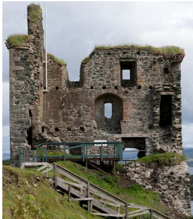
Tower house internal elevation
