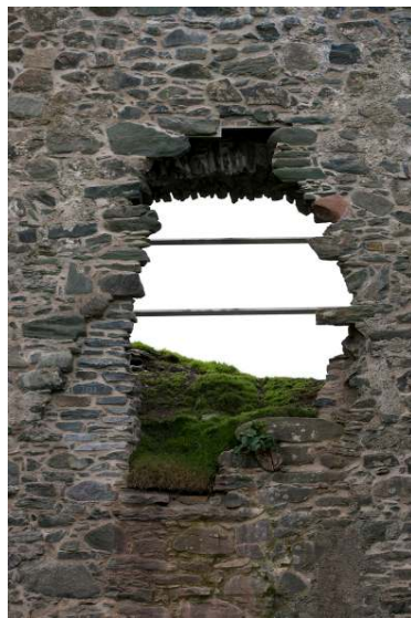
First floor N window (O)
