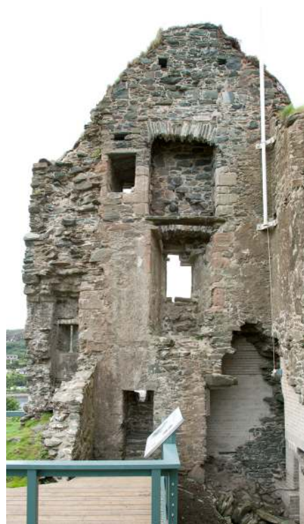
Tower house internal elevation
